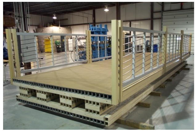
The SCB was constructed off-site with a modular design using layers of square composite tubes.
